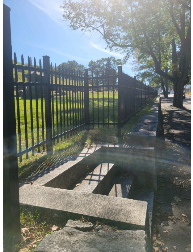
Laurel Hill Fence Replaced
